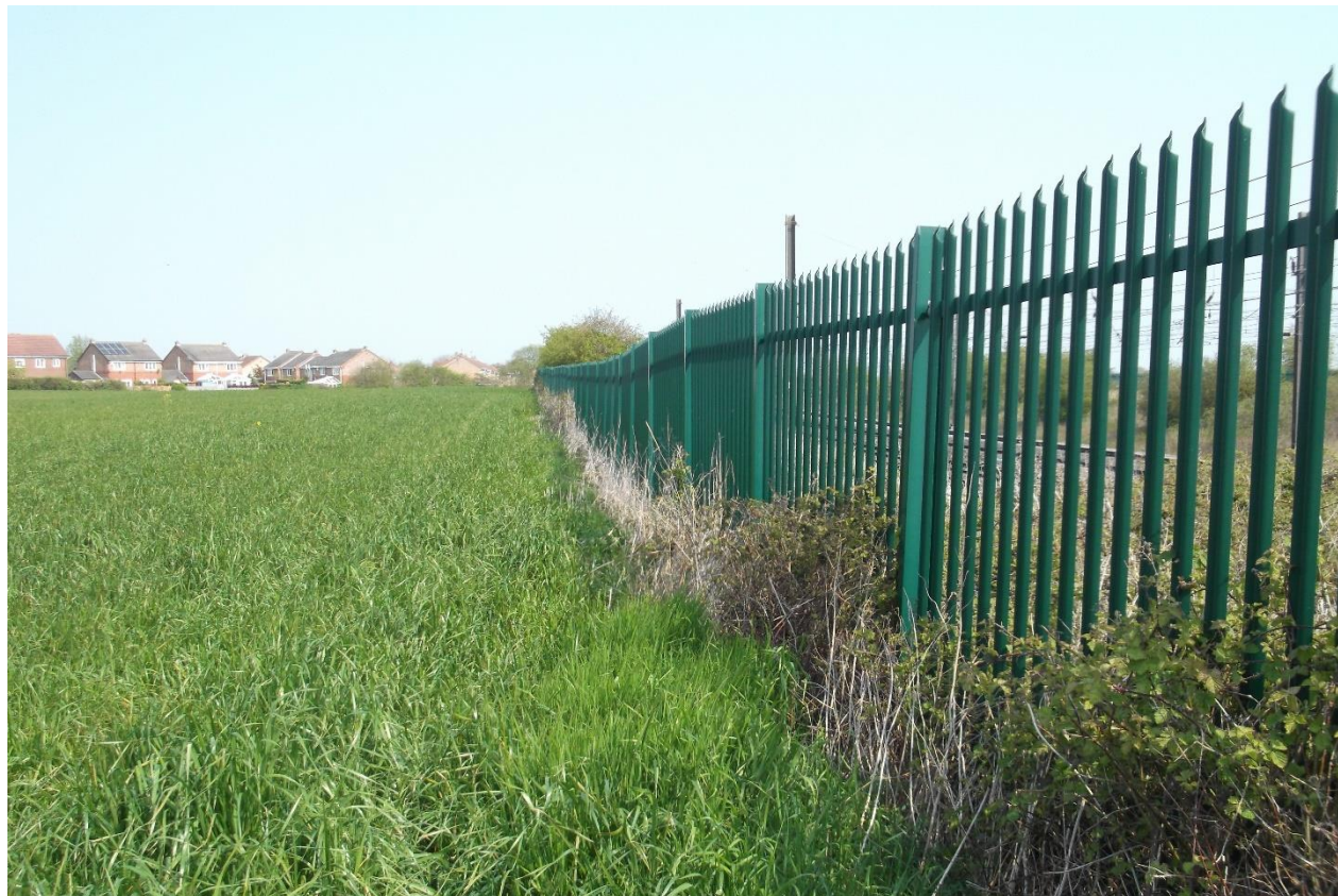
Site Boundary with Railway Line
